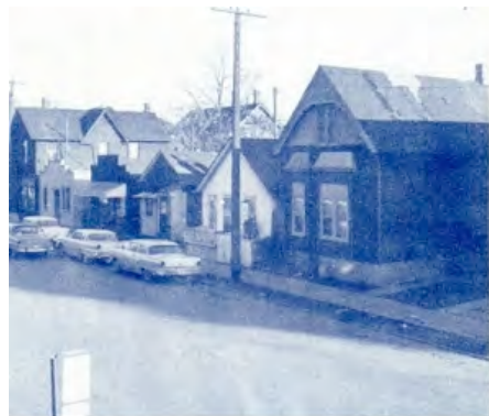
Detroit -- West Side Industrial Typical Conditions -- Before
